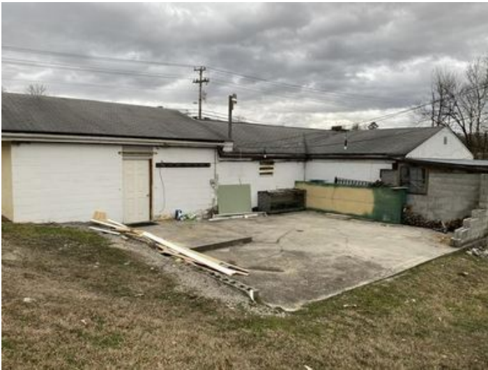
2. Back of building
